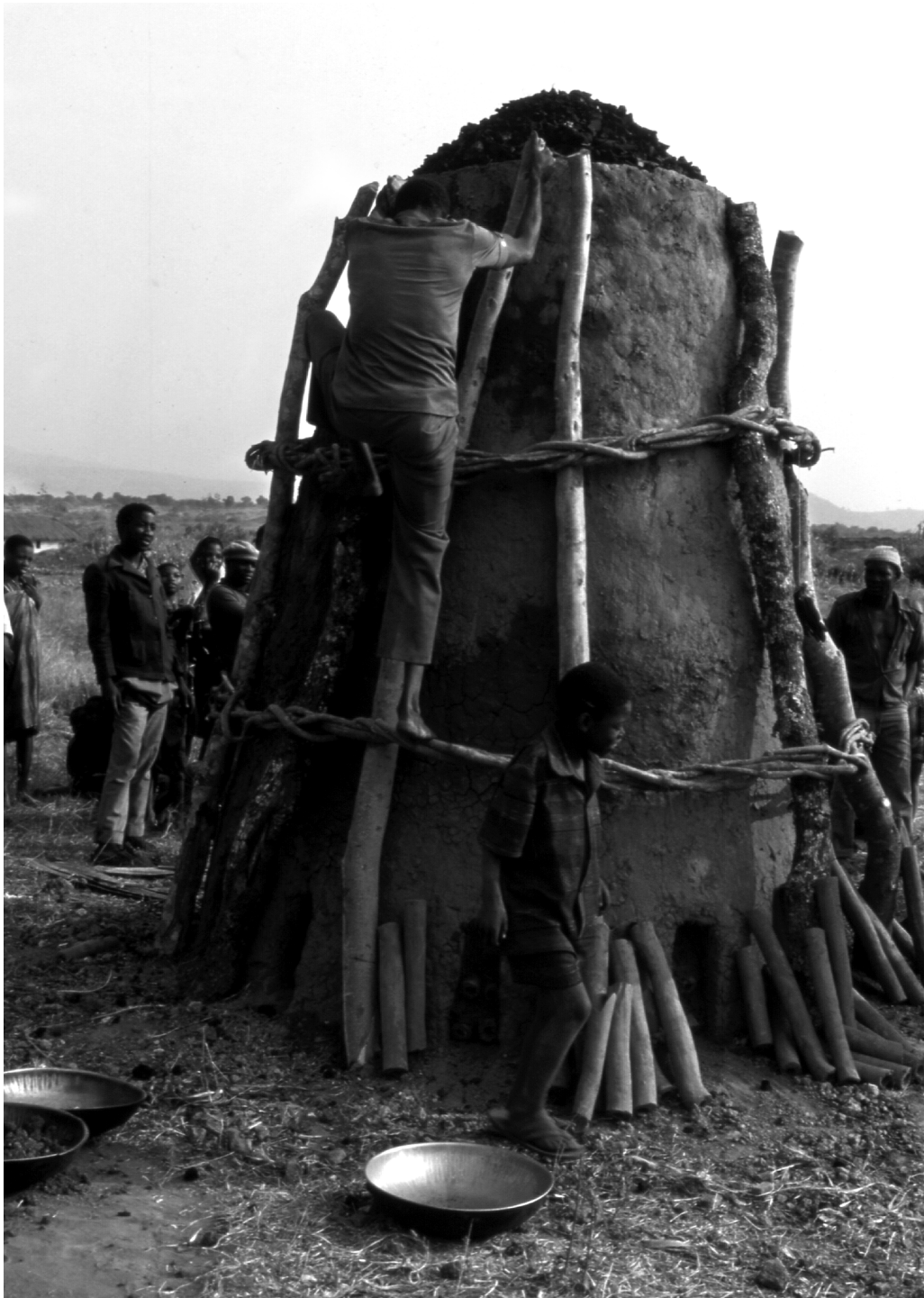
Fig. 5. The large furnace is made ready for smelting among the Fipa. Photo R. Haaland.
